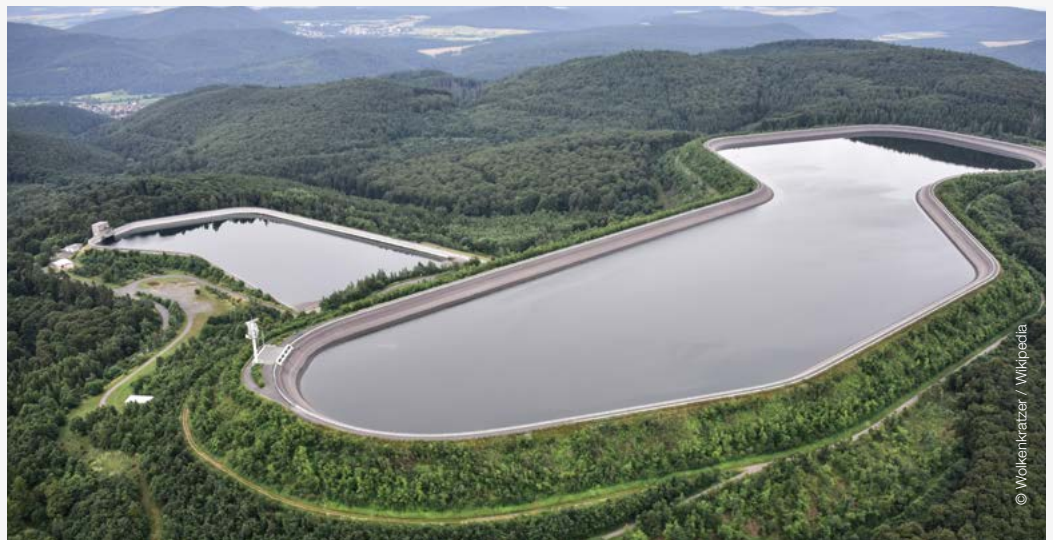
Uniper Kraftwerke GmbH / Germany has installed the systems in PSPP Waldeck 1 (one 70 MW pump turbine) and Waldeck 2 (two ternary units each 240 MW) in 2017
