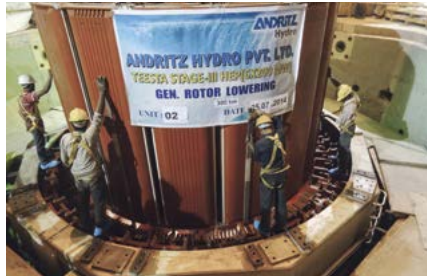
Generator rotor lowering
