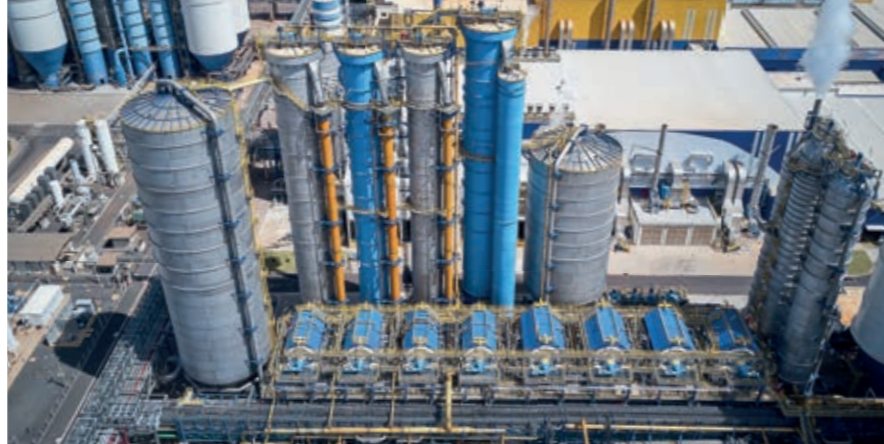
The new hardwood fiberline ensures low operating costs, low emissions, extremely high washing efficiency, and excellent fiber quality. The capacity (6,120 adt/d) is the highest in the world for a single fiberline.
