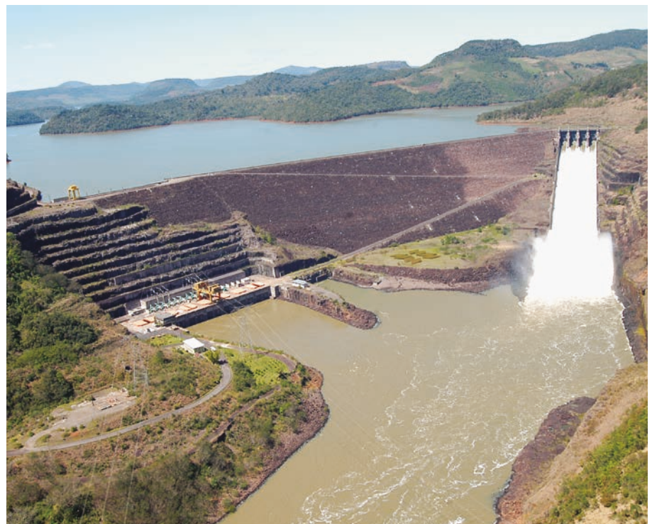
Downstream view of power house, dam and spillway
