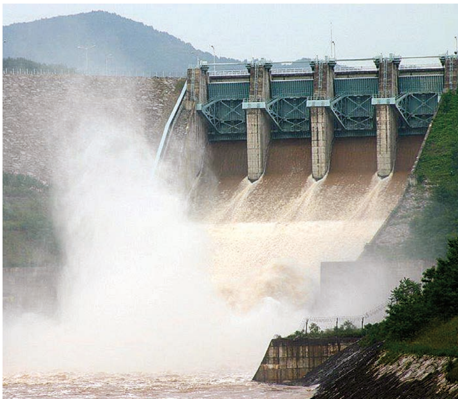
Dam and spillway
