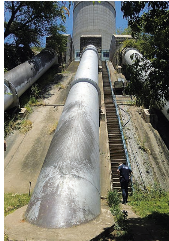
Penstocks before rehabilitation works
