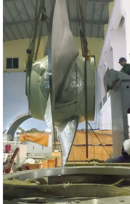
Runner installation at HPP Chi Khe
