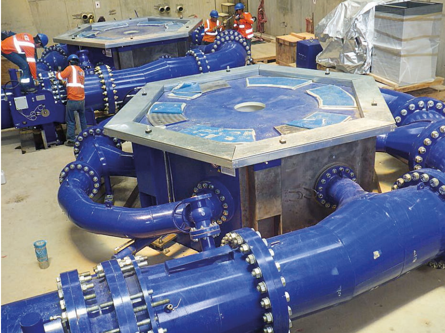
Installation works at HPP El Carmen
