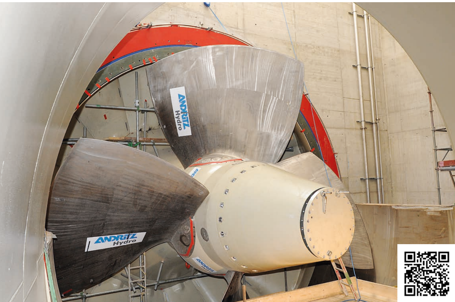
Bulb turbine runner during installation process at HPP Iffezheim, Germany
