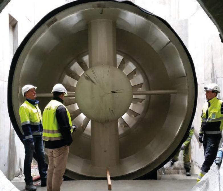
Installation works for a small Bulb turbine
