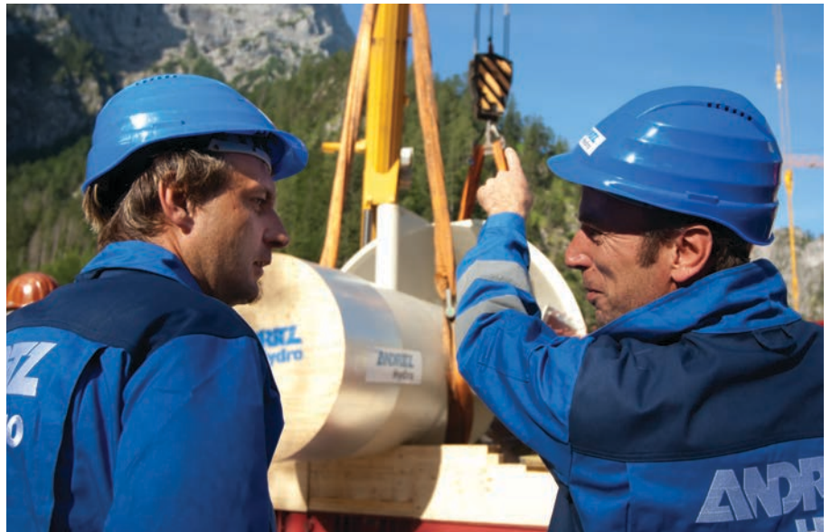
ANDRITZ HYDRO team during Bulb turbine installation
