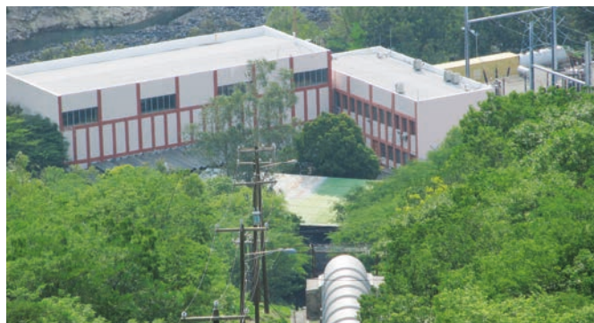
Powerhouse and existing penstock of HPP Carlos Fonseca
