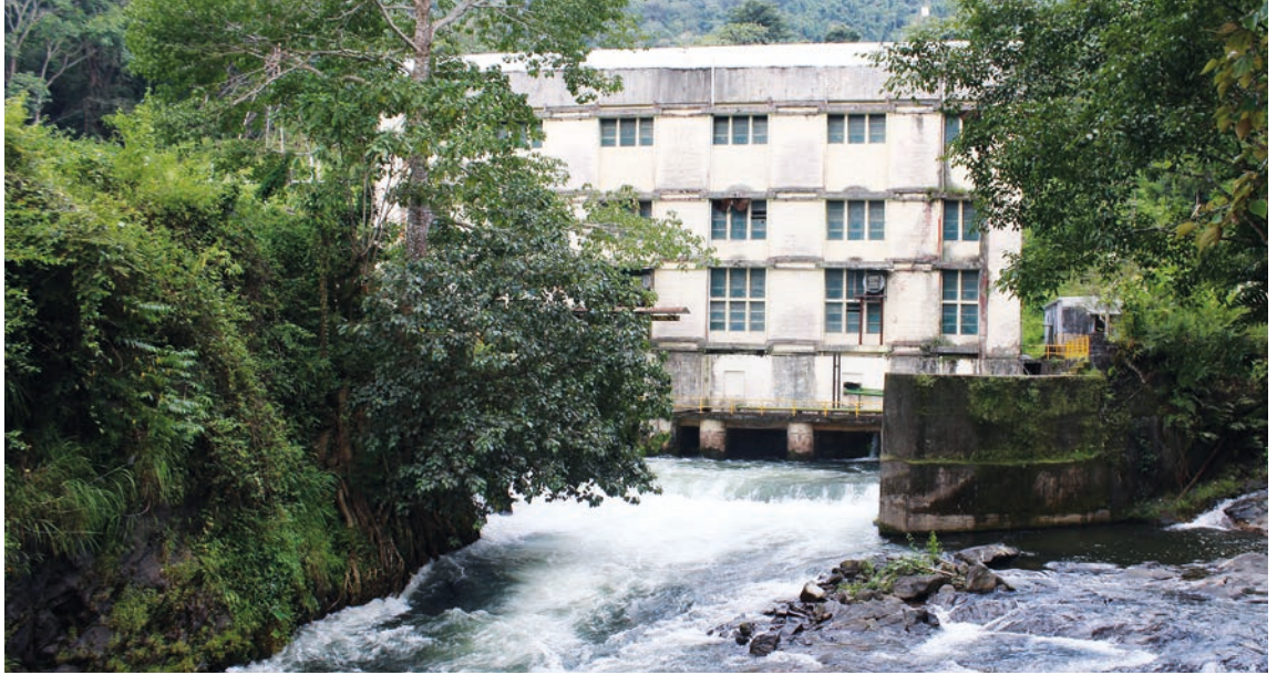
Power house and Sholayar River
