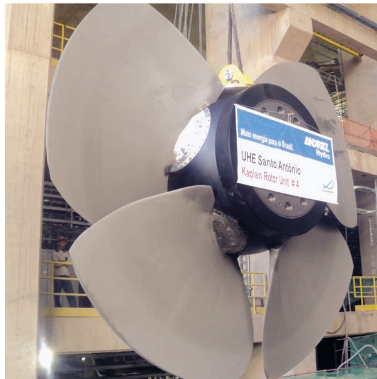
Installation of Bulb turbines at HPP Santo Antônio, Brazil
