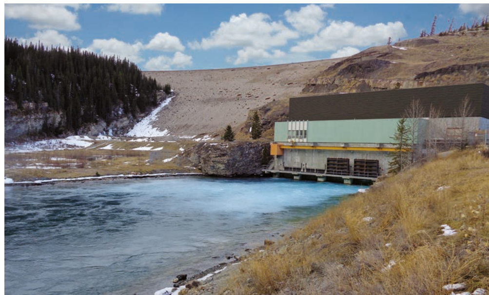
Downstream view of the site and dam
