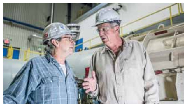
Russ Lang, Supervisor (left), with Rinus Jellema, Steam Plant Superintendent in front of the new turbine. ▶
