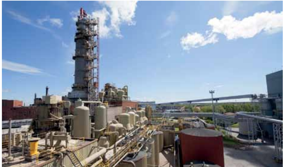
▲ The Veitsiluoto complex includes a sawmill, pulp mill with energy production unit, and paper mill. Annual output from the pulp mill is 375,000 tonnes of both hardwood and softwood pulp (swing production). The first OPE contract was for cooking, brownstock washing, and the evaporation plant.
