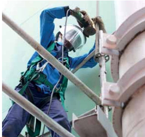
◀ Maintenance on the fiberline.
