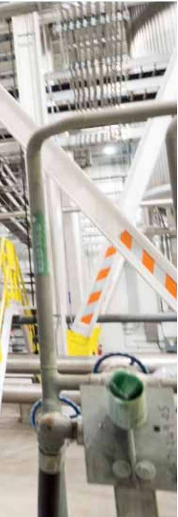
◀ The scrubber vessel's waste ash pickup point, including the fluidizing air ring and ash transport lines.
